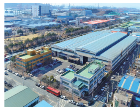
Noksan Office and Factory
